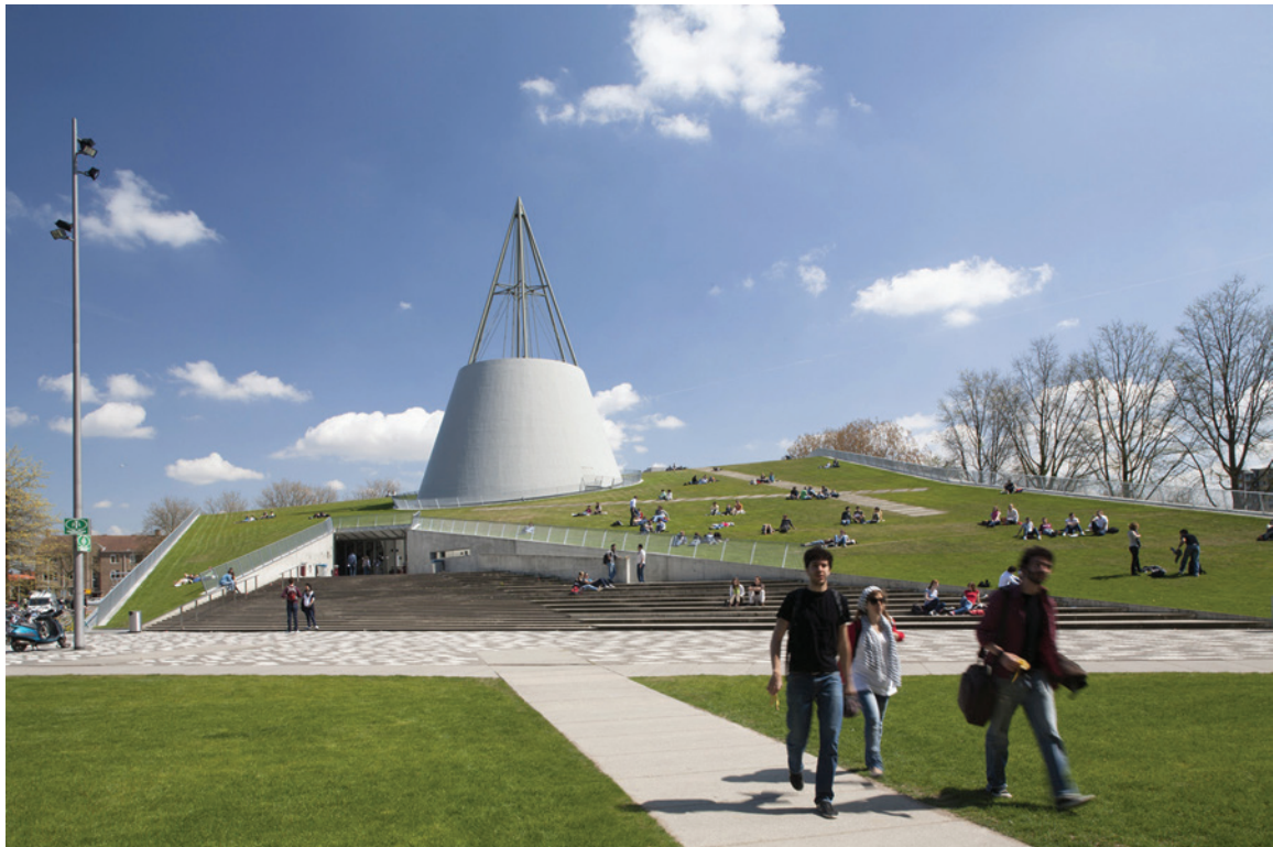
Fig. 4: Students taking advantage of the green roof.
