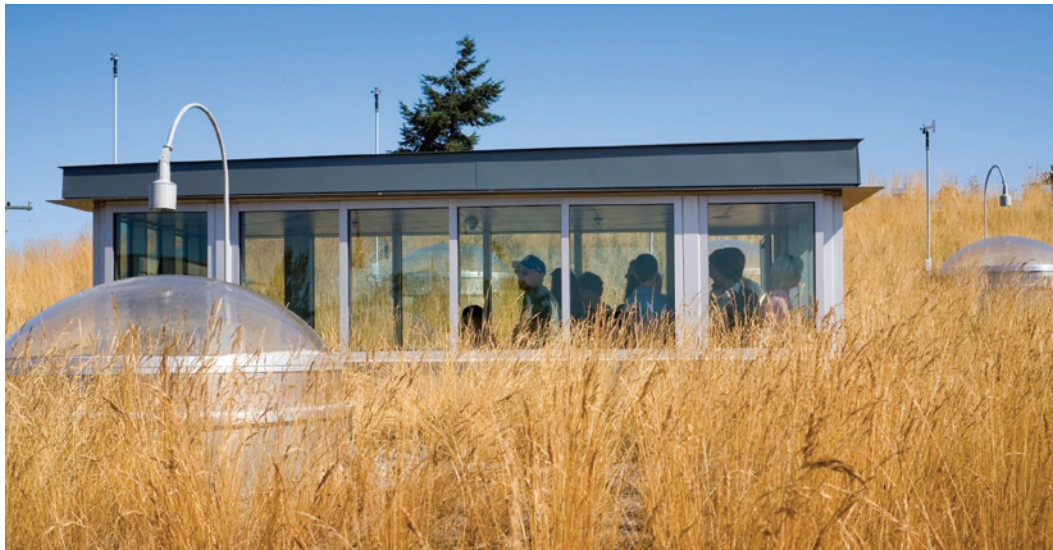
Fig. 7: Lookout on the green roof
